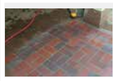
Tile and Grout Cleaning
